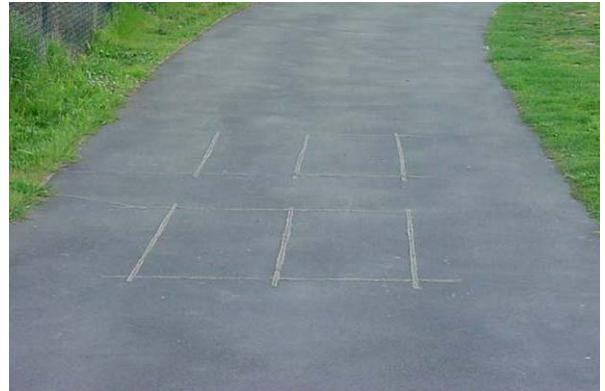
Now a little high-school or college physics is necessary to introduce the principles involved; bear with me... A low current is fed through the wire loops, which in turn produces an electromagnetic field (EMF) that ‘orbits’ around the wires. If you hold your left hand in a “hitch-hikers pose” (i.e. clenched with thumb out) then, if the current in the wire is travelling in the direction of your thumb, the EMF is circulating in the direction of your other fingers.
