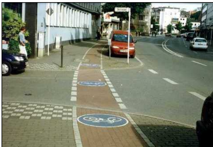
Figure 1: Poor intervisibility but clearly delineated pathway at side street
