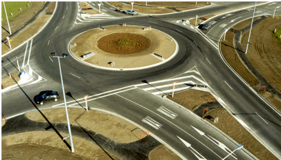
A recent roundabout reconstruction in Christchurch (Bexley/Dyers). Note the handrails at all crossing points.
