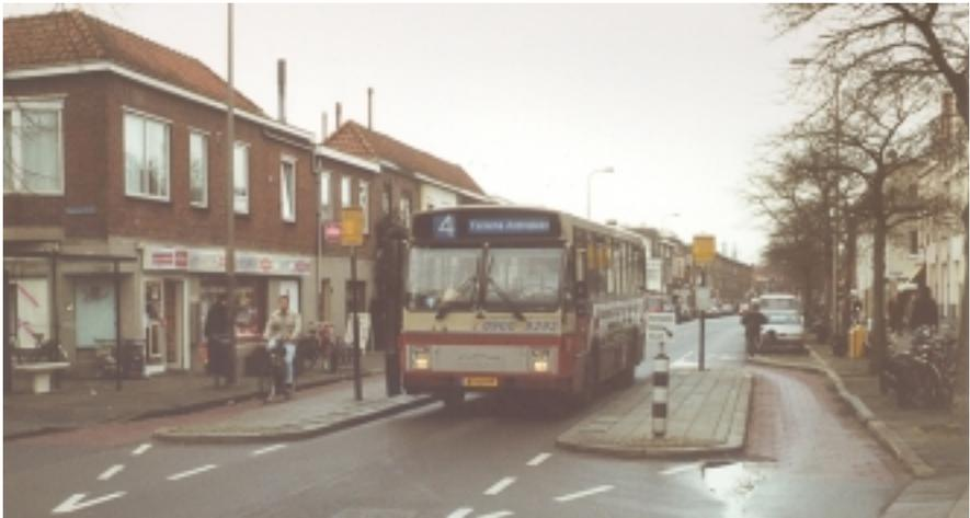
This is a busy shopping street, parked cars line the kerbs, visibility for pedestrians is reduced. To keep traffic moving at a safe speed single width "squeeze points" are employed, to avoid cyclists getting squashed bypasses are provided. Need a bus stop? Build it on the traffic calming so that when a bus stops so does all the traffic. Should a child run out behind this parked bus it won't be struck by a passing car. Simple, effective.
