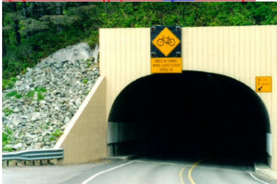
Figure 1: 'Share the Road' Promoted by Signage at Tunnel Entrance 1
