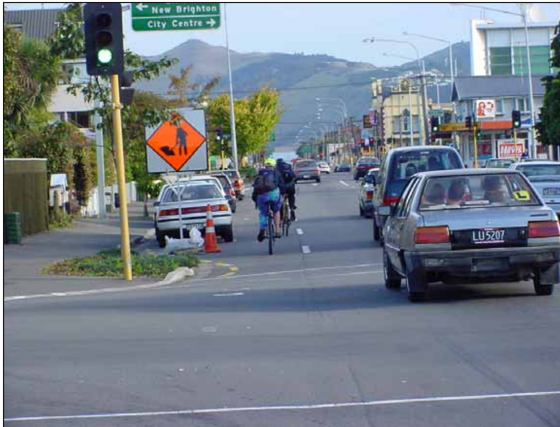
Figure 1: Considerate placement of a roadworks sign at the edge of a shoulder, leaving an appropriate passage for cyclists without forcing them into the traffic lane 1 .
