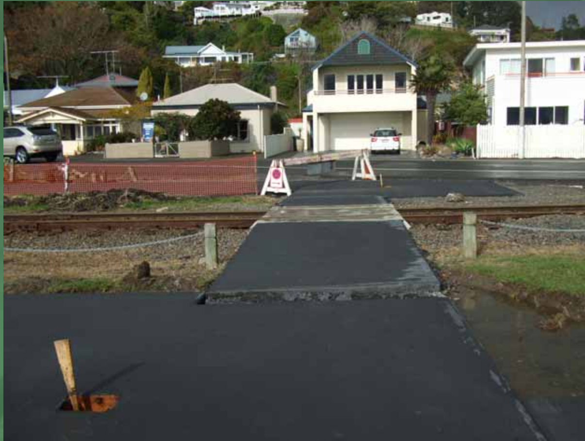
Rail level crossing at western end during construction
