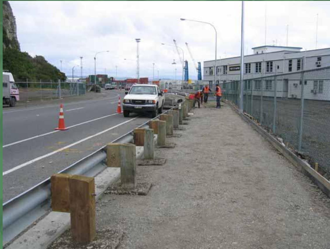
Guardrail installation at chainage 600m
