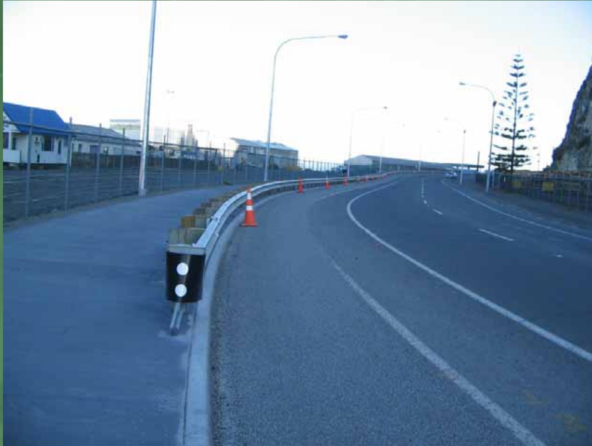
Completed guardrail end terminal
