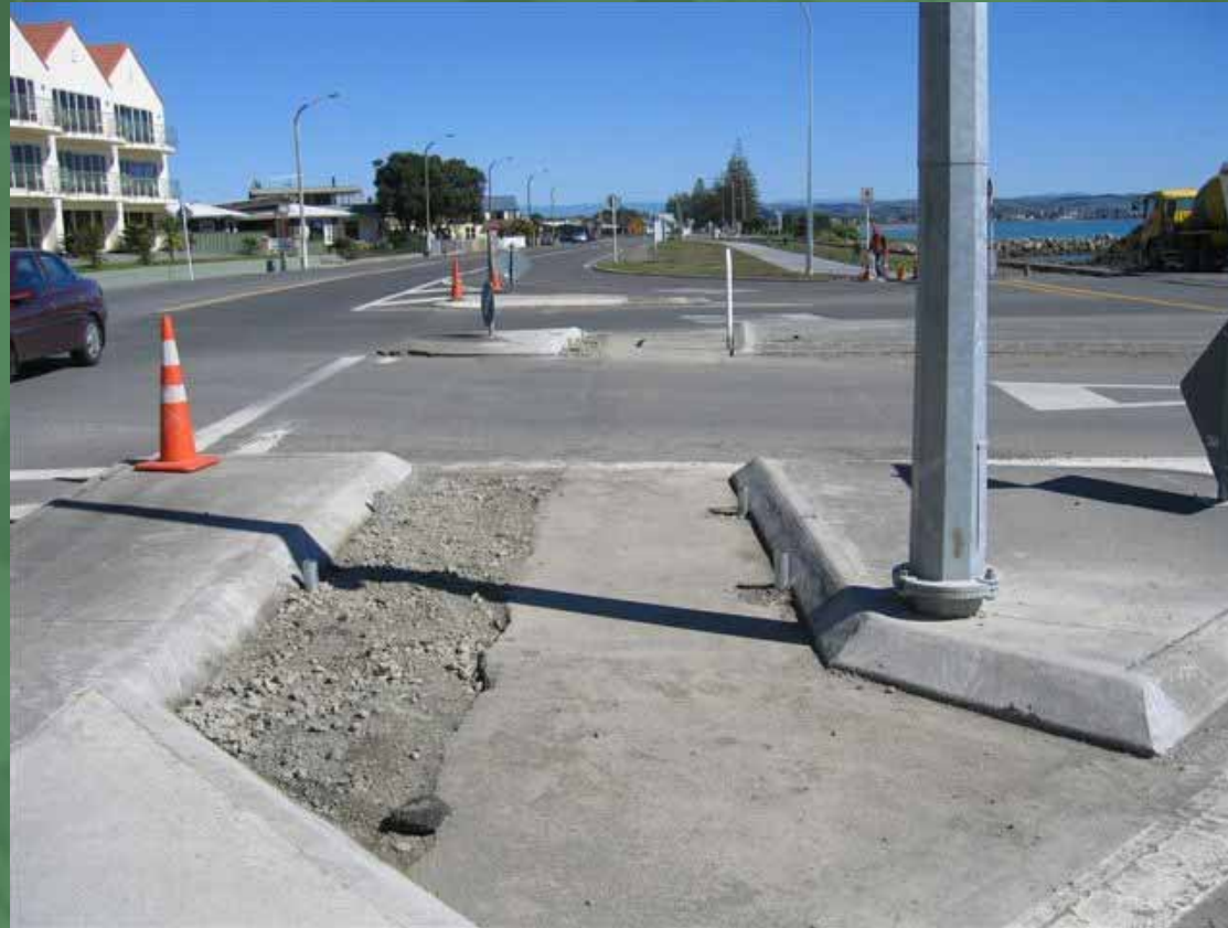
Gate 3 heavy truck entry into Port of Napier pedestrian & cyclist crossing
